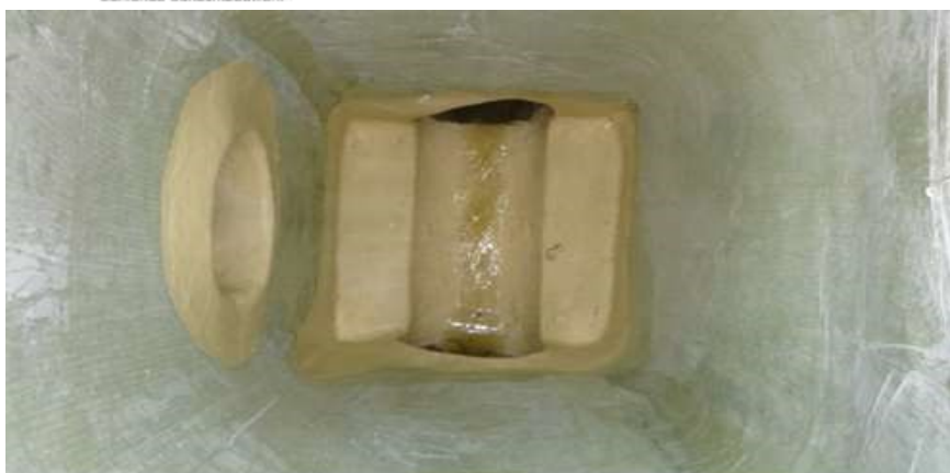
Figure 14. Renovimi i pusetave
