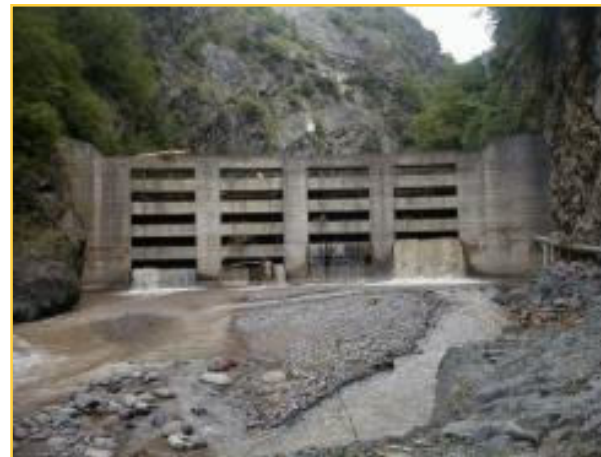
Filtering check dam
