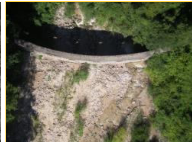
Retention check dam
