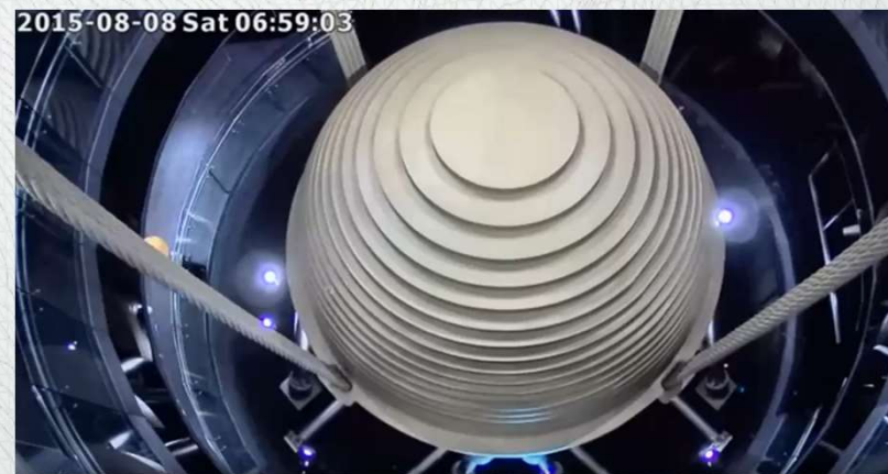
Tuned Mass Dampers (TMD) – Taipei 101 Tower – Taipei - Taiwan
